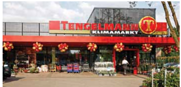
The high heat insulating properties of OKAGEL insulating glass supports the innovative, energetic concept of the climate market. The building needs only 50 % of the energy required by comparable markets and has zero CO 2 emission.
