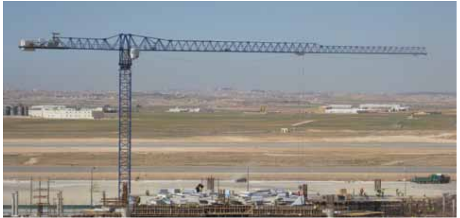
Extension of the Amman's International Airport in Jordan by LINDEN COMANSA
