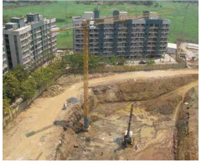
Liebherr 71 EC-B 5 FR. tronic Flat-Top crane in the field
