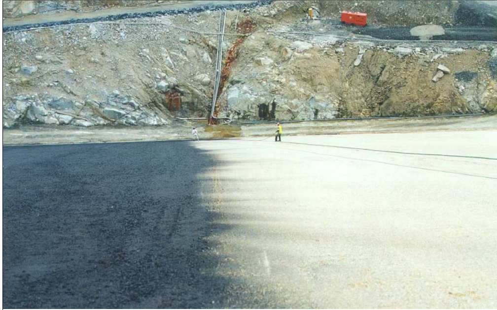
La Galaube Dam- Upstream face - July 2000 Impregnation with bitumen emulsion
