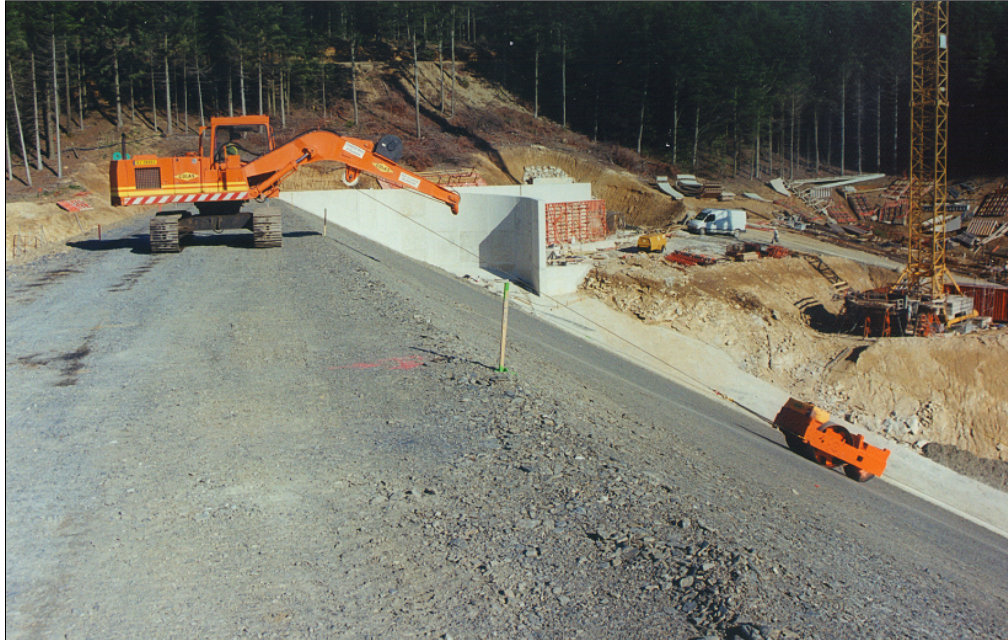
La Galaube Dam Compaction of backfilling - July 2000
