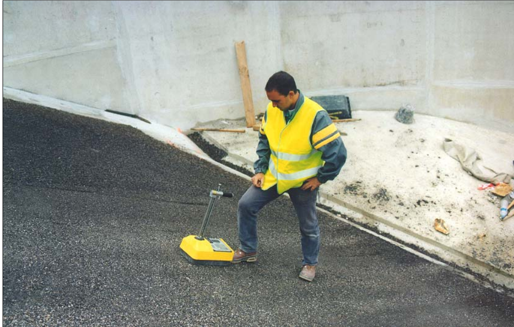
La Galaube Dam- August 2000 Control of compaction of cold asphalt 0/10
