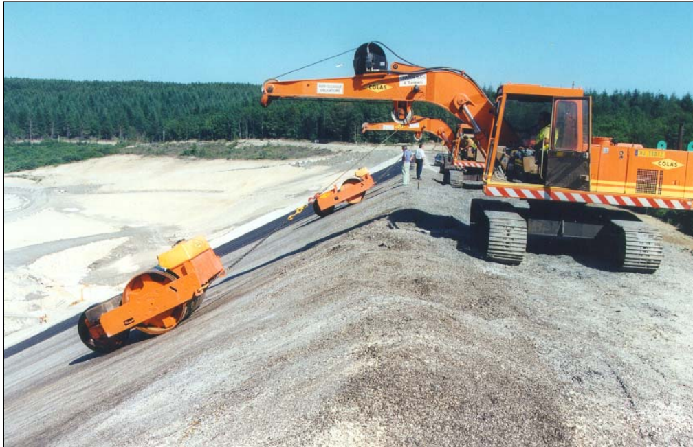
La Galaube dam- August 2000 Compaction of cold asphalt 0/10
