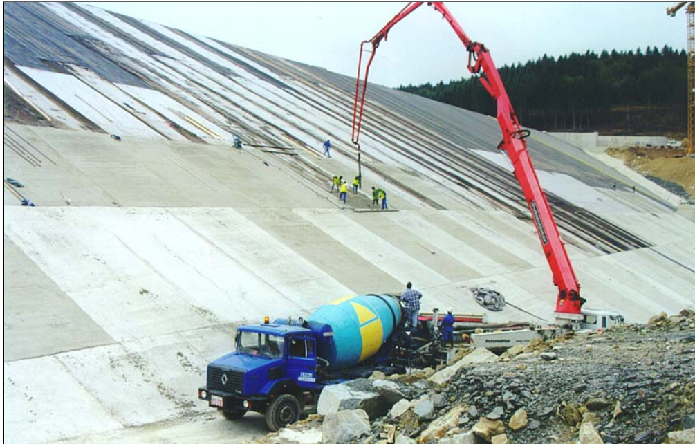
La Galaube Dam - October 2000 Laying concrete on the top of Coletanche
