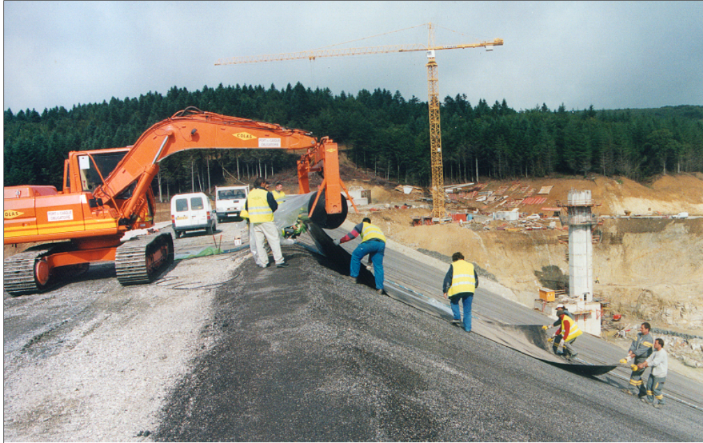
La Galaube Dam- September 2000 Laying COLETANCHE NTP3
