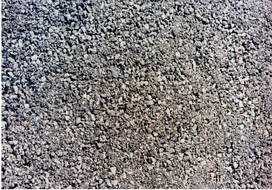
La Galaube dam - August 2000 Surface aspect of cold asphalt 0/10
