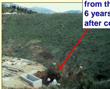
VALCROS DAM DOWNSTREAM SLOPE
