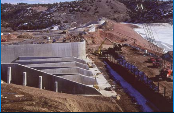
Steel Sheet Pile Installation
