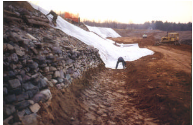
Figure 6. Installation of upstream geotextile seepage barrier
