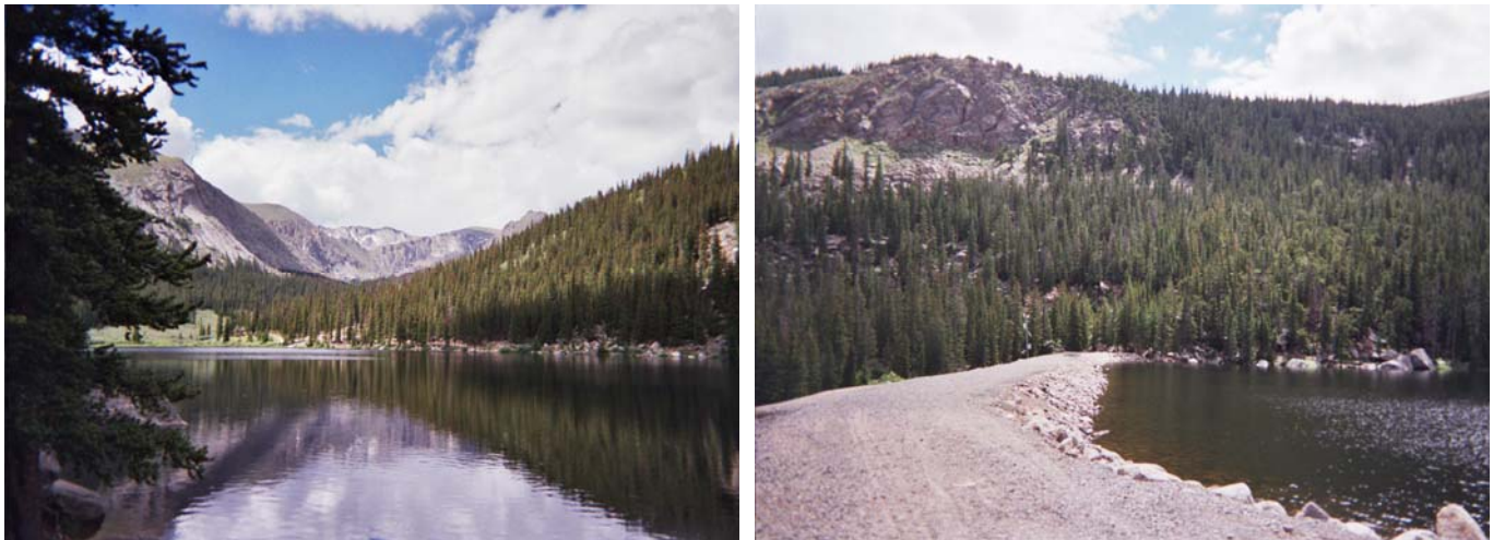
Figures 1a and 1b. Idaho Springs Reservoir and Dam.
