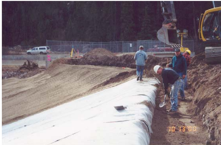
Figure 3. GCL Installation
