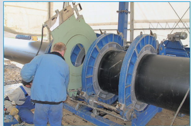
Figure 3 Heated tool but welding
