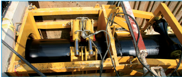
Figure 1 Swagelining tool to reduce diameter
