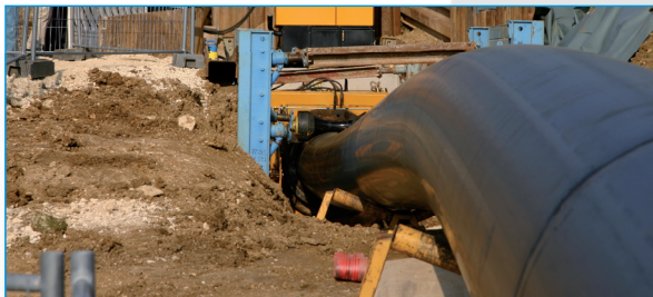
Figure 2 Pull in of the pipeline with OD 900 mm
