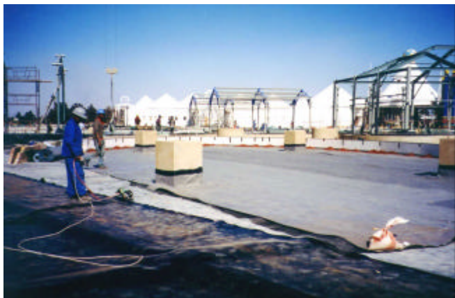
Photo 2: Carnival City - Lining of Water feature
