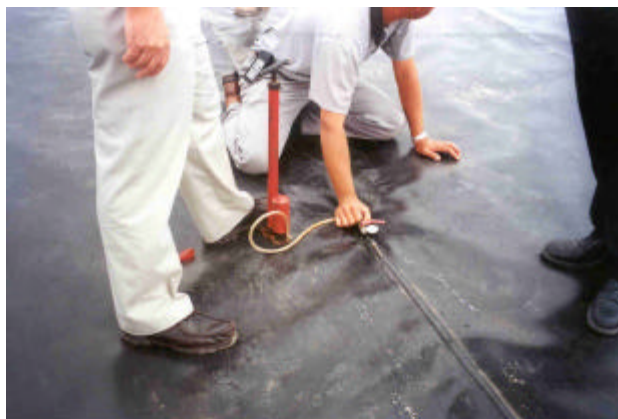
Photo 4: Testing of Double Wedge Weld
