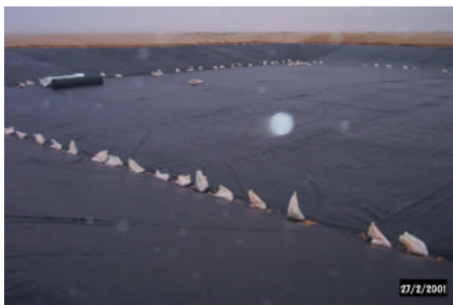
Photo 3: Walvis Bay Hazardous Cell Secondary Liner
