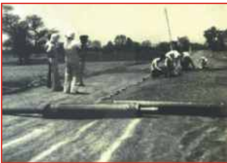
Geotextile laying
