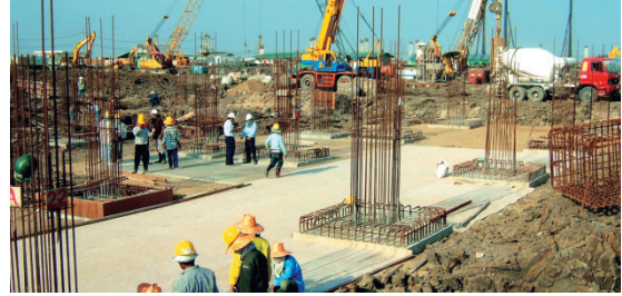
Thailand Waterproofing of an airport hotel
