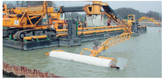
Germany Underwater installation in a canal lining system
