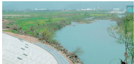
Japan Flood protection dam
