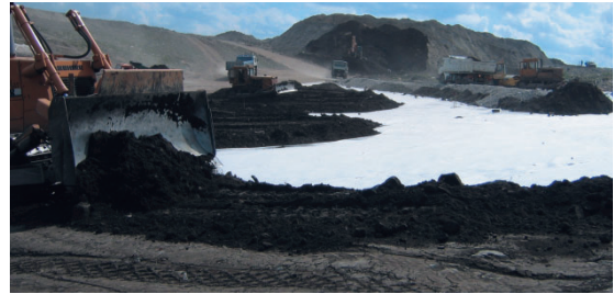
Estonia Landfill capping with Bentofix® and Secudrain®
