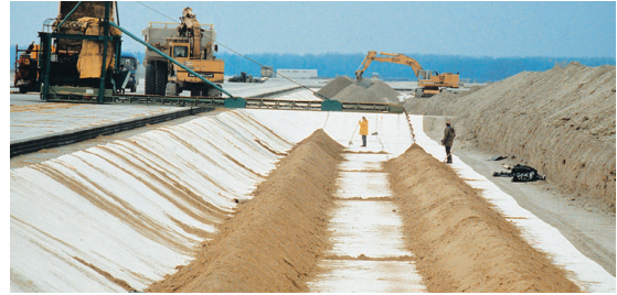
Germany Sealing of Airport runways
