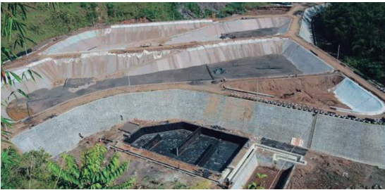
Bali Landfill base sealing with Bentofix®
