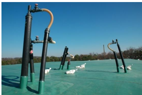
Boot Fittings and Flashing Details
