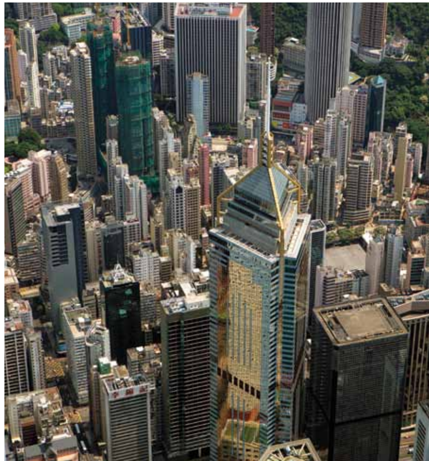
Aerial view overlooking Wanchai, Hong Kong.
