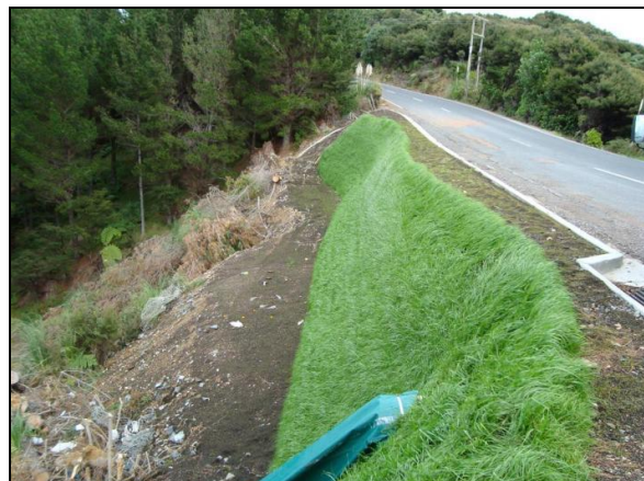
(c) Permanent vegetation established on the compost-sock facing of the slope.
