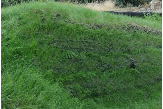
(f) Vegetated, sock-module MSE wall several weeks after completion.
