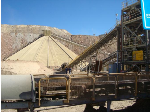
Heap leach mining liner
