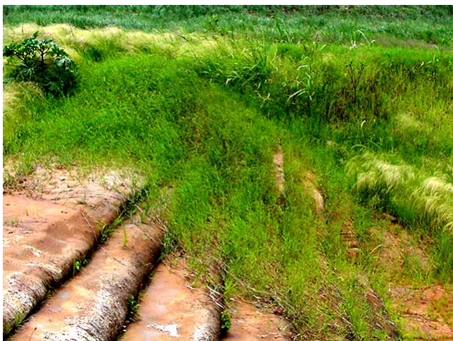
Close-up view of a tier of Geo steps, showing Vetiver grass taking over.
