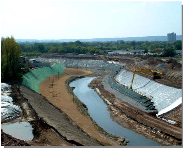
GCL use in Canada: Rennie Street Landfill, in Hamilton City, on Lake Ontario. Composite liner using a GCL to line a waterway through the landfill.
