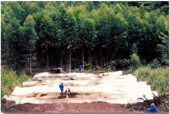
Flexmesh being laid over the wetland, before placing of dumprock
