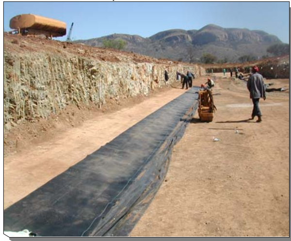
Placing of 1.0mm HDPE liner (Hidriline) on canal floor after excavations
