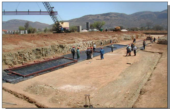
Preparation for concrete on floor of canal over 1.0mm Hidriline
