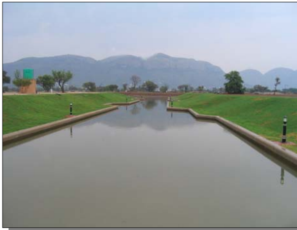
Northern view of completed phase 1
