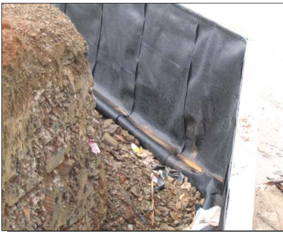
canal walls Extended view of HiDrain drainage layer on
