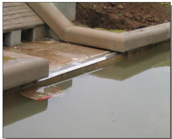
Detail view of HiDrain drainage layer on outside of
