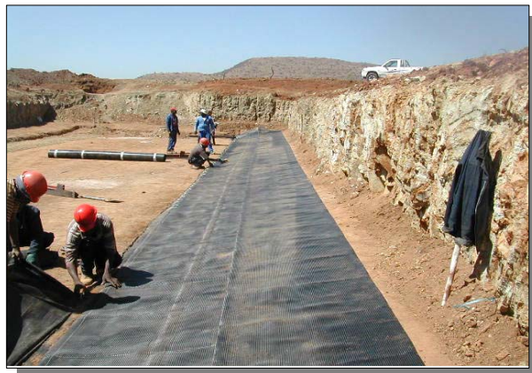
Closer view of Hidriline liner and excavations
