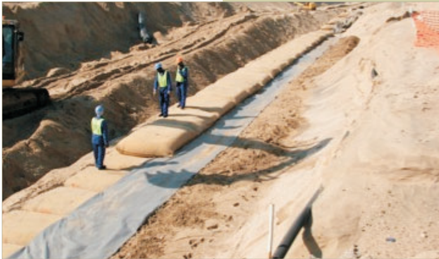
Photo 2: Single Layer of EnviroRock™ with RockGrid® PC wrap around wall
