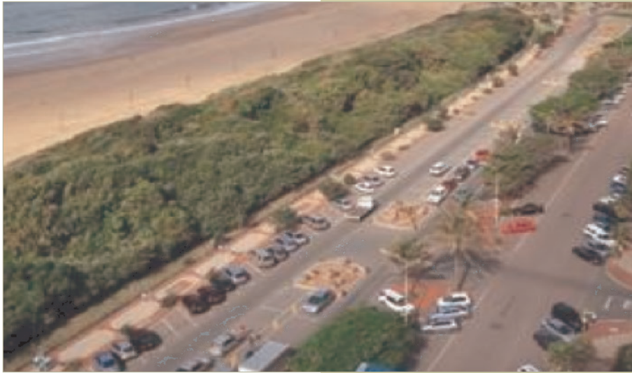
Photo 1: Aerial View of the Durban Promenade
