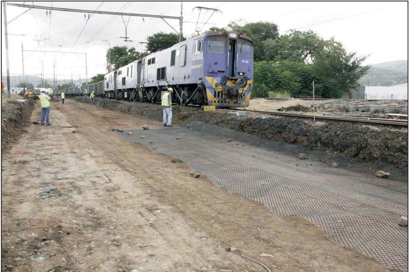
TriAx® being laid on the Kaapmuiden turnout
