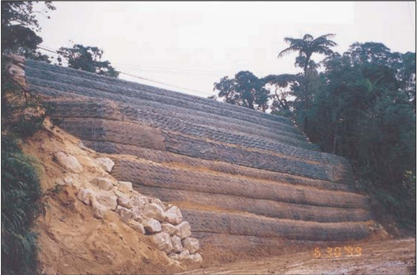
Figure 3 : Reinstatement of the slope
