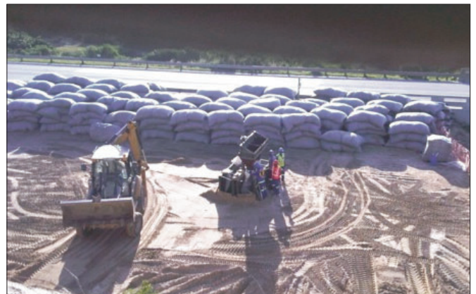
Stockpiling of sand-filled bidim geocontainers
