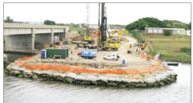
Completed eastern platform
