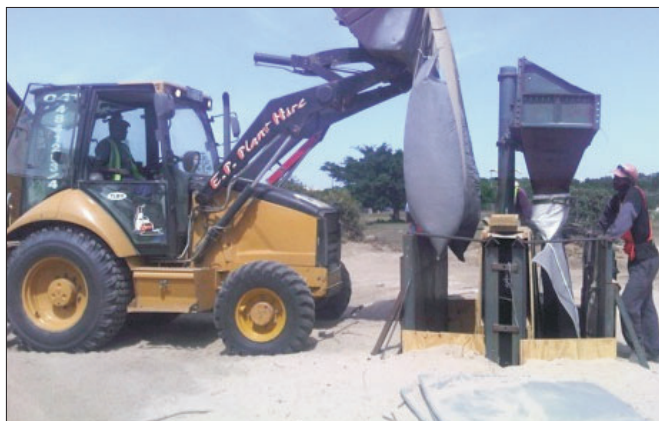
Geocontainer filling operation
