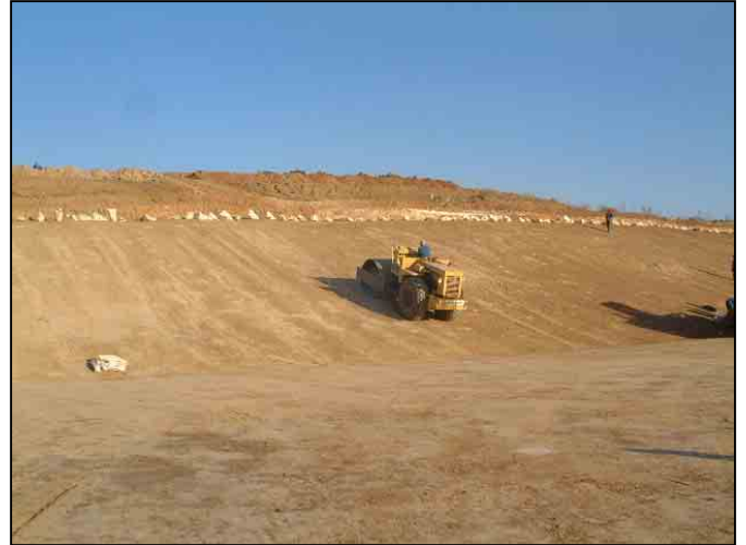
Photo 2: Compaction of the clay layer
