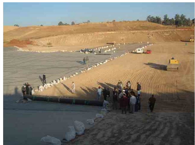
Photo 3: Installation of HDPE geomembrane liner
