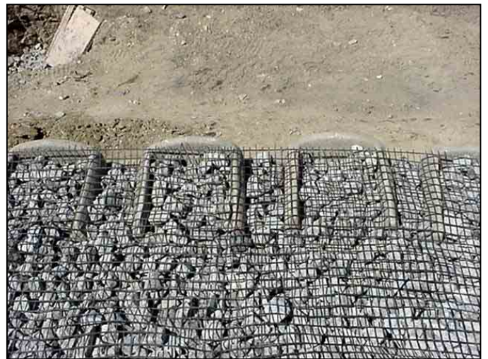
Photo 2: Rock GX Geogrid in place
