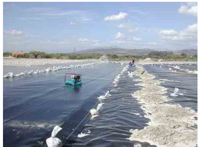
Figure 3: LLDPE liner at central drain of Cell 1
