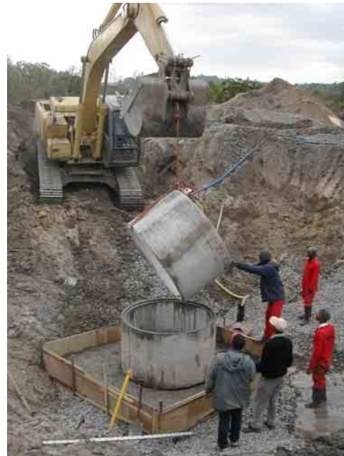
Figure 2: Construction of subsurface drainage pump station for leachate pond
