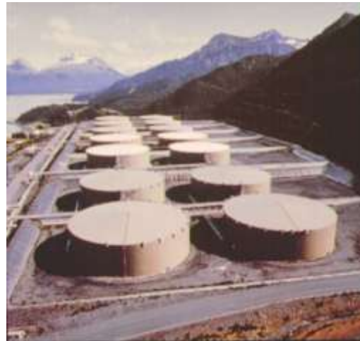
Figure 3. Geomembranes used as secondary containment for tank farms, gas stations, etc.
