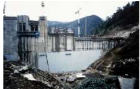
(c) Roller compacted concrete dam
