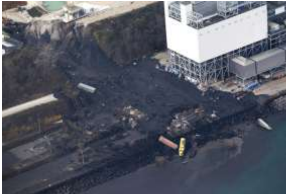
Figure 4. Recent failures of dry and wet disposal of coal combustion residuals.
