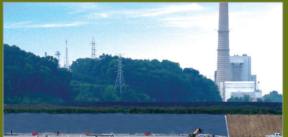
COAL ASH DISPOSAL
