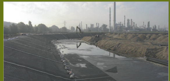
HAZARDOUS WASTE & CHEMICAL STORAGE
