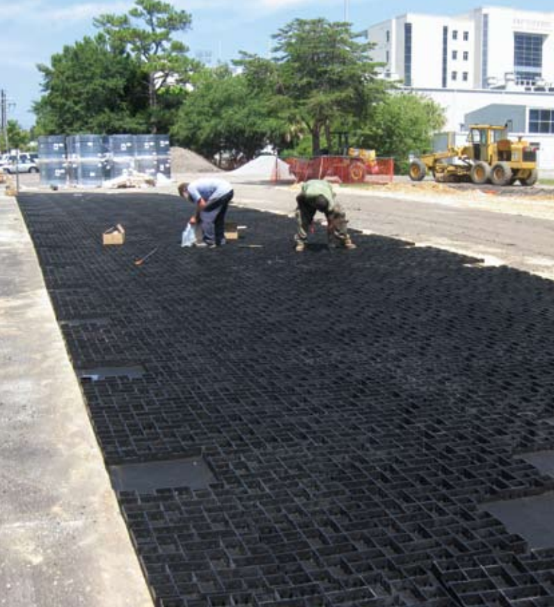
Crews place GeoPave units on a mesh bottom (left). At right, the cells are ready to be filled with aggregate.
