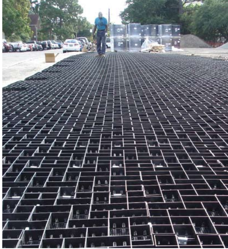
Crews place GeoPave units on a mesh bottom (left). At right, the cells are ready to be filled with aggregate.
