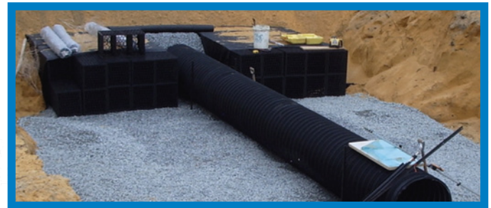
LANDSDALE ROAD SYSTEM during construction showing gross pollutant collection pipe.
