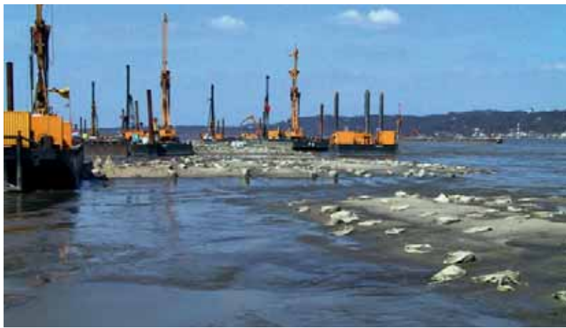
Embankment foundation with Ringtrac® system geotextile-encased columns
