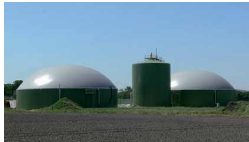
Double-membrane roof for biogas plants
