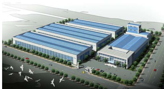
Great Vision - Xinzhuang New factory - - Geomembrane (under construction )
