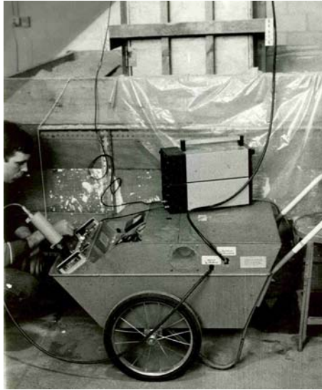
Figure 2 – Continuous wave microwave unit designed and manufactured in the Drexel University nondestructive evaluation techniques research program by Koerner and Lord (c1980).
