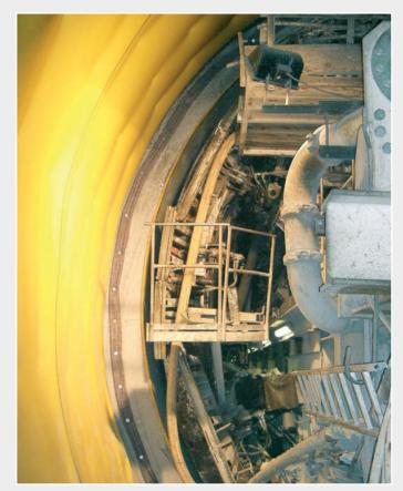
The finished welded sealing layer before concreting the inner shell of the tunnel.
