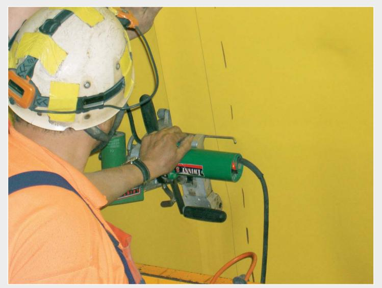
The TWINNY S can be easily guided, even in the case of vertical weld seams.
