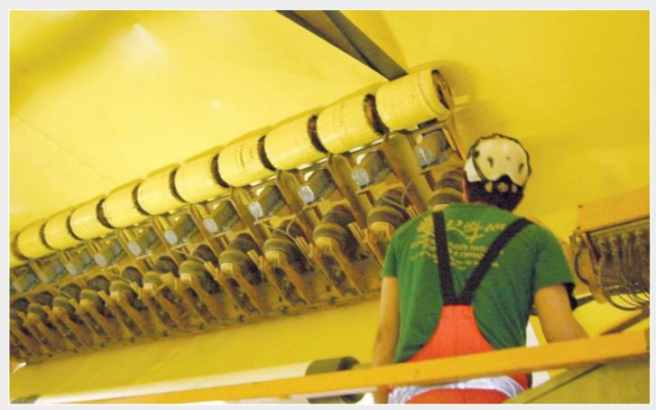
Mechanical application of the prefabricated, 14 ft wide plastic sealing sheets onto the Velcro-backed discs located below. Welding is then carried out.
