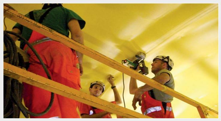
Overhead welding work with the TWINNY S.
