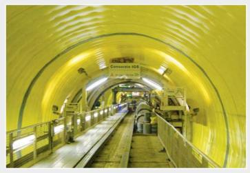
Finished tunnel seal. The individual sheets are welded in parallel.
