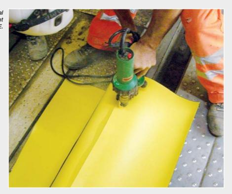
"Double" pressure roller and welding nozzle of the TWINNY S.
