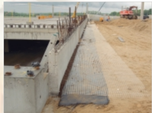
Secugrid® reinforced "soil pressure absorber" in front of the cellar wall
