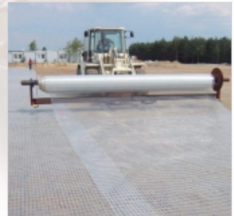
Secugrid® installation
