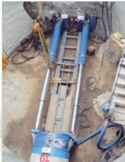
Feeding of a Carbofix® sealed pipe in the shaft
