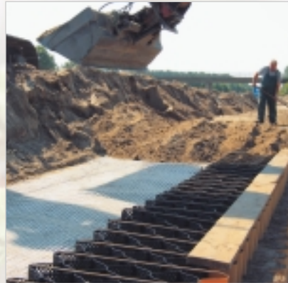
Filling of the Secugrid® reinforced geocells
