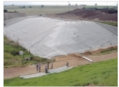
Installation of 1.5 mm Carbofol® geomembrane
