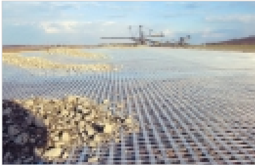
Secugrid® 100/100 Q6 before being covered using a former overburden excavator
