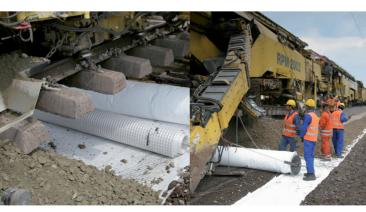
underneath the rails, screening, cleaning of the ballast and FPL (Frost Protection Layer), installation of the filtration/separation geotextile and reinforcement geogrid, and installation and compaction of the new FPL and ballast layers. For the third section, work was performed through more conventional methods.
