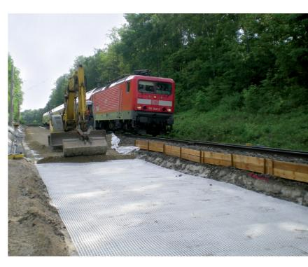
of cover soil. Secugrid<sup>®</sup> geogrids are also manufactured in accordance with the EBA's guidelines.
