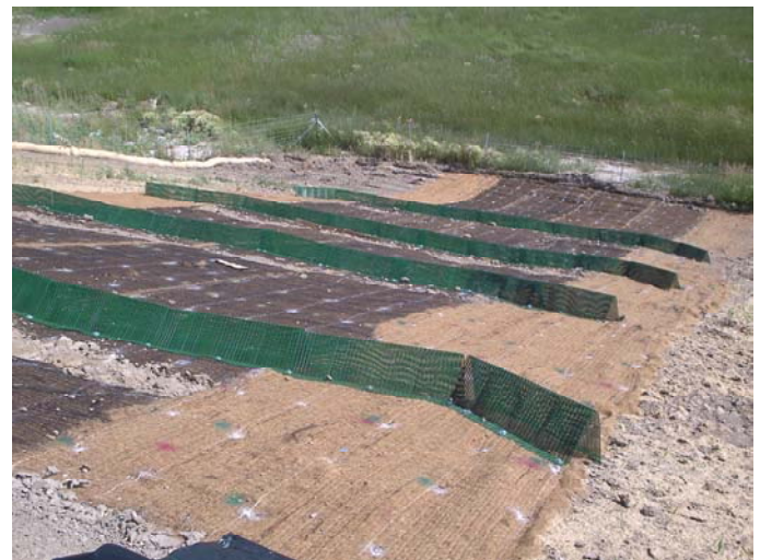
E-470 Off Ramp – Colorado Installed on coconut and straw coconut blanket
