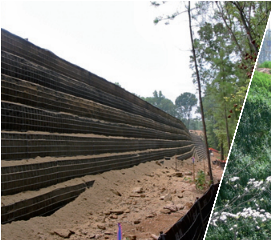
The retaining wall after construction
